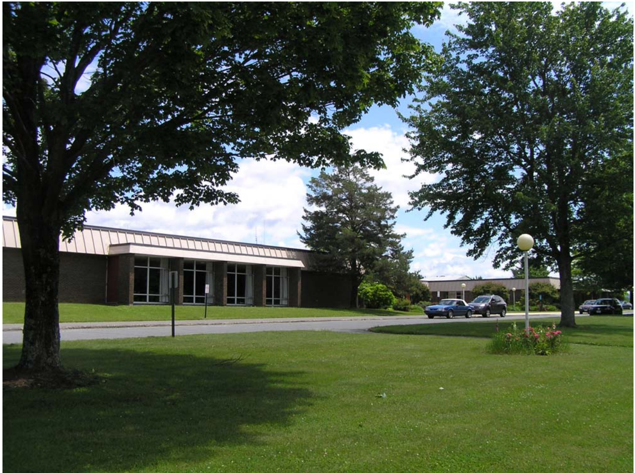
(Existing Monument Mountain Regional High School)
